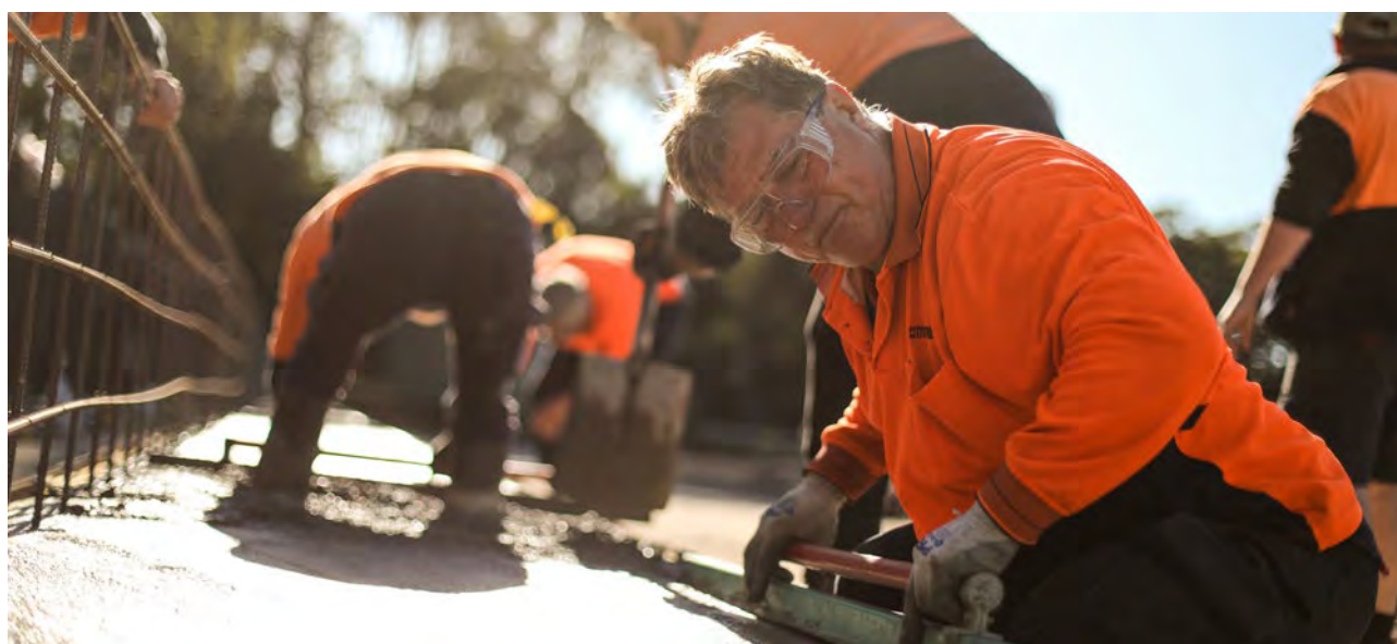
Image: Council staff renewing a footway
